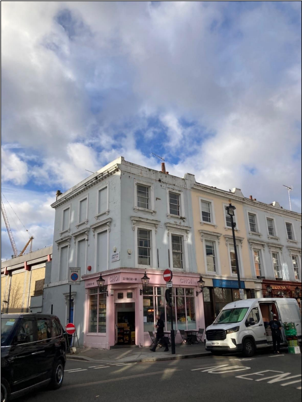
22 Upper Tachbrook Street
