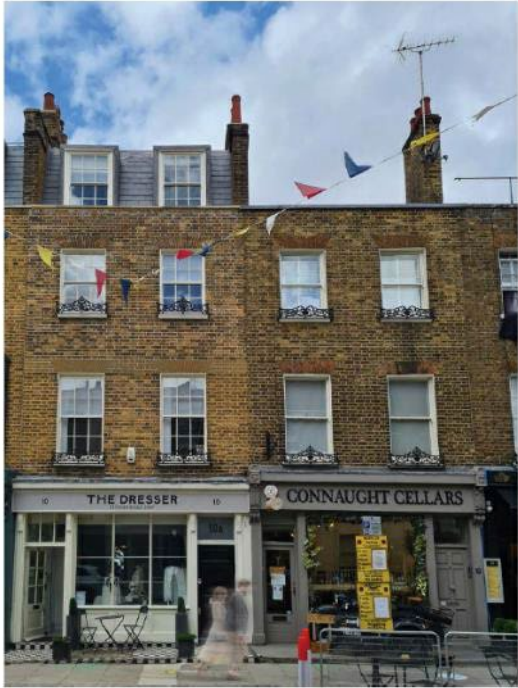
Existing shopfront at 8, Porchester Place (Connaught Cellars)
